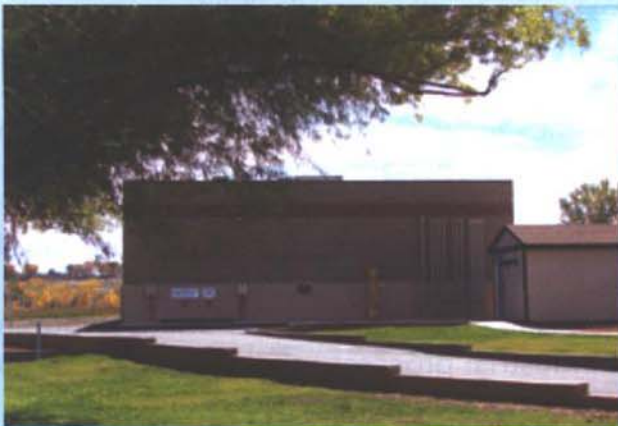
New pre-treatment facility
